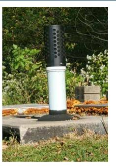
The unique design of the odor control canister allows for a quick installation and simple filter changing operation.
